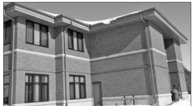
Operators Local 139 training site Coloma, WI.
